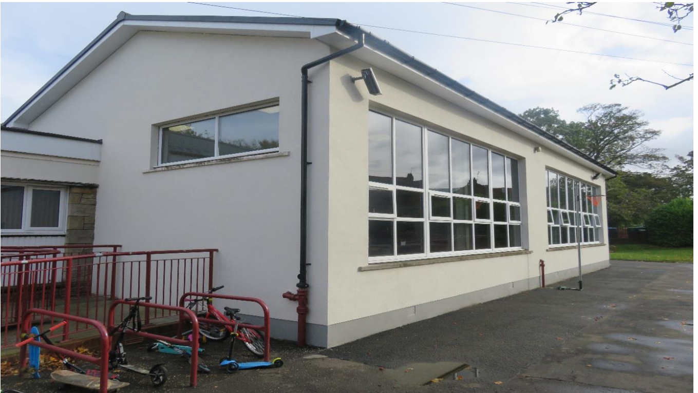
Photograph of External Wall at St. Margarets PS after Enhancements
